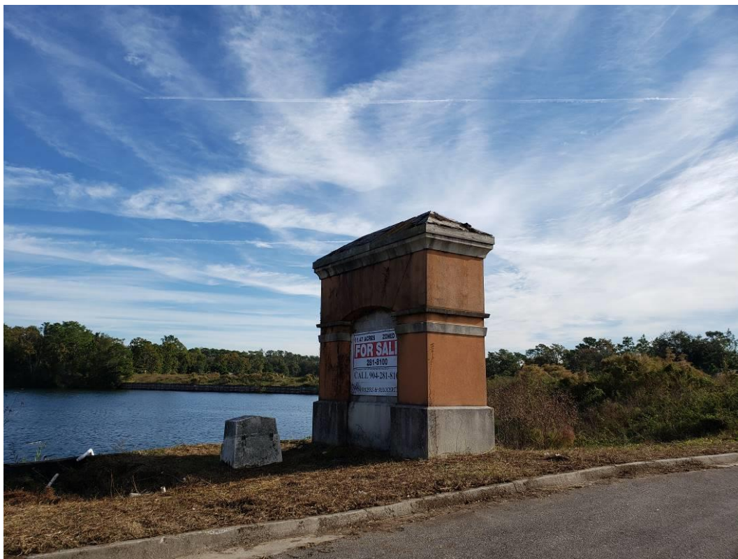
Existing monument sign next to entrance road
