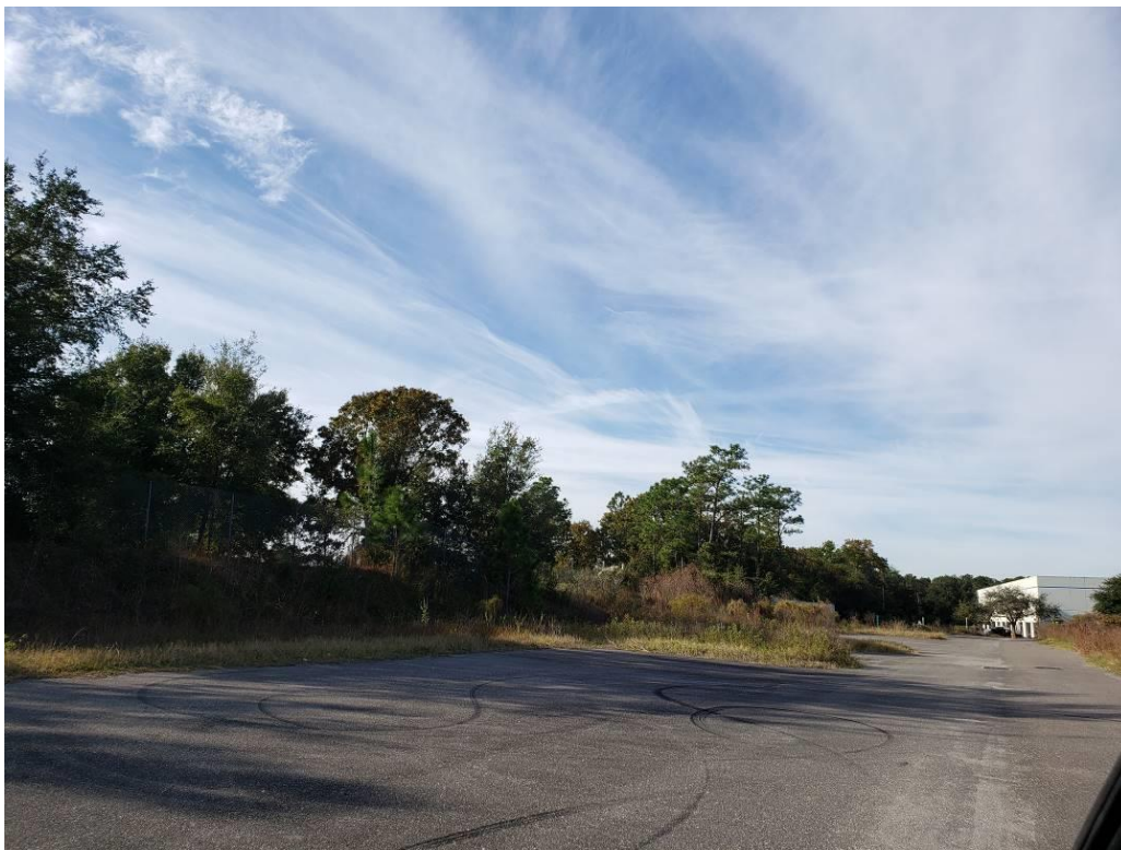
Existing roadway on site, with unpainted parking area
